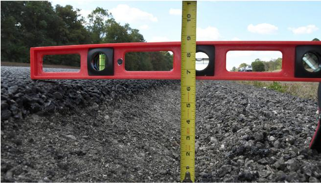
**Figure 3** - Shoulder drop-off due to construction activities.
