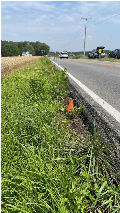
**Figure 4** - Roadside drop-off due to lack of maintenance.
