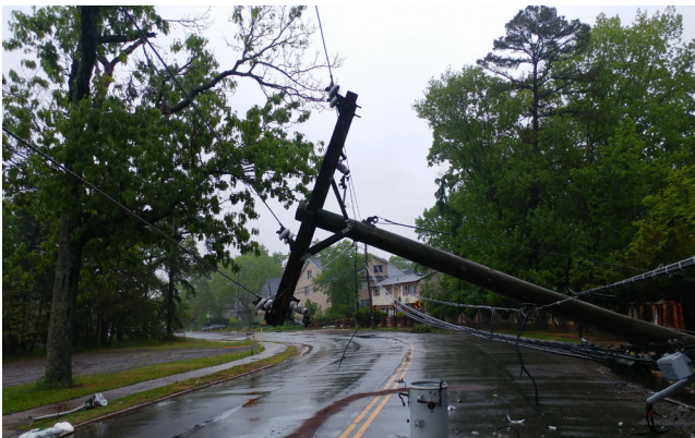
Figure 6 - Downed power lines resulting from a severe storm and high winds—common damage following tornadoes and hurricanes in the Southeast.
