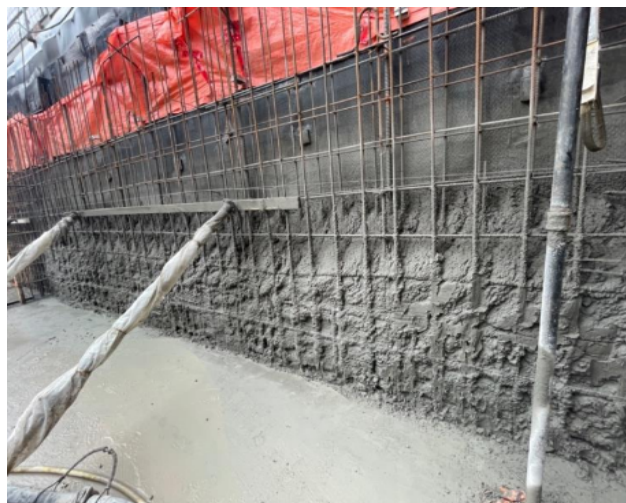
Figure 3 – Use of shotcrete for foundation wall construction.
