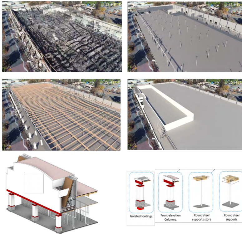
Figure 5 - LIMS - virtual reconstruction of a property affected by a fire event.
