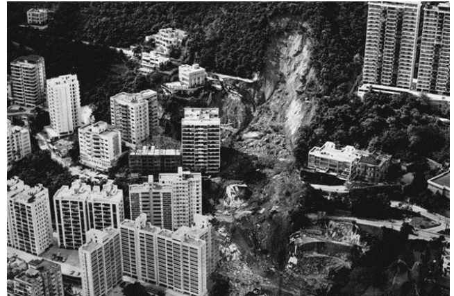
Figure 6 - 1972 Po Shan Road Landslide in Mid-Levels of Hong Kong that toppled a 12-story building and caused 67 fatalities (Source: https://www.scmp.com/magazines/post-magazine/short-reads/article/2098525/deadly-1972-twin-landslides-hong-kong-claimed ).
