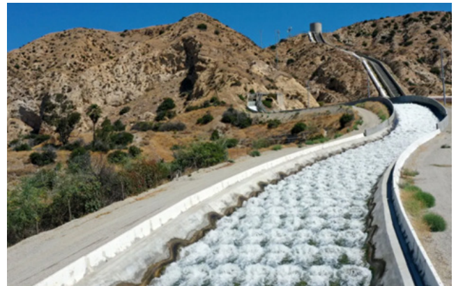
Figure 5 - Water flows down the Los Angeles Aqueduct, relying on the geometry of the landscape to gravity flow down toward the City of Los Angeles
