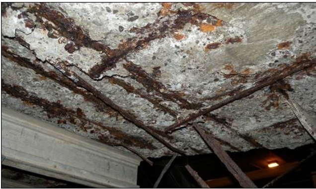
Figure 3 - A close-up of the underside of the concrete slab shows the severe corrosion of reinforcement rebars.
