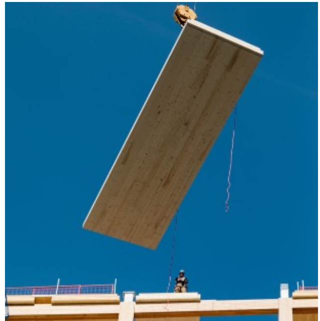
Figure 2 - CLT mass timber floor panel installation during construction.
