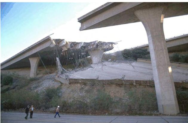
**Photo 3** - A destroyed segment of the I-5 Freeway in Northridge, California; 1994 (Credit: [FEMA/Wikimedia Commons](#))
