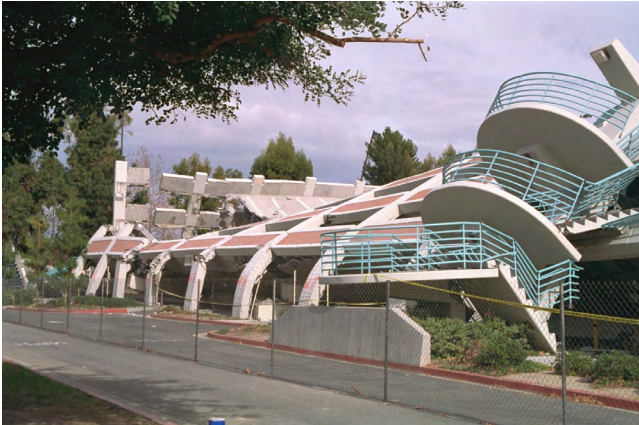
Photo 4 - Structural collapse of a five-year-old parking garage in Northridge, California; 1994. (Credit: USGS archive )
