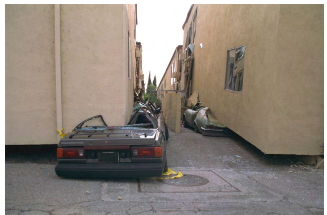
Photo 2 - Soft story collapse resulting in crushed vehicles, (Credit: USGS archive )
