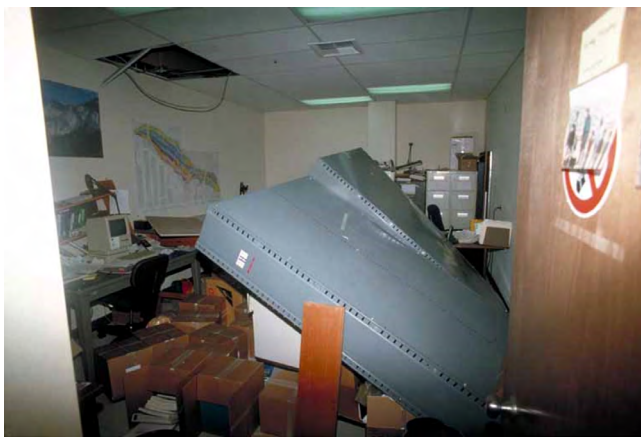
Photo 1 - Heavy bookcases, boxes, and shelving toppled during an earthquake (Credit: USGS Denver Library Photographic Collection )
