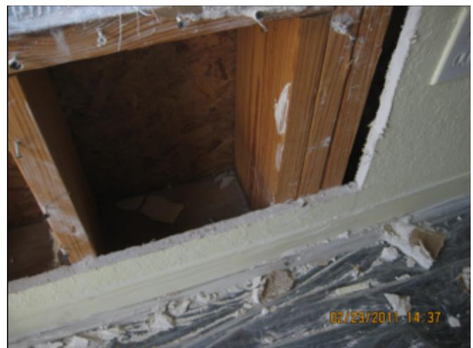
*Figure 3 - Destructive Testing performed on interior face of wall*
