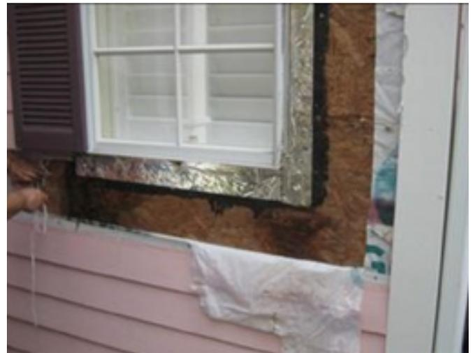
*Figure 6 - Limited deconstruction below window*
