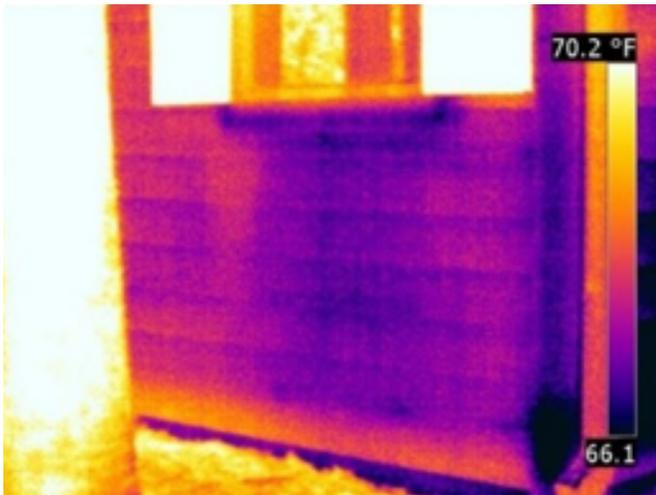
*Figure 5 - Thermal anomalies below window*
