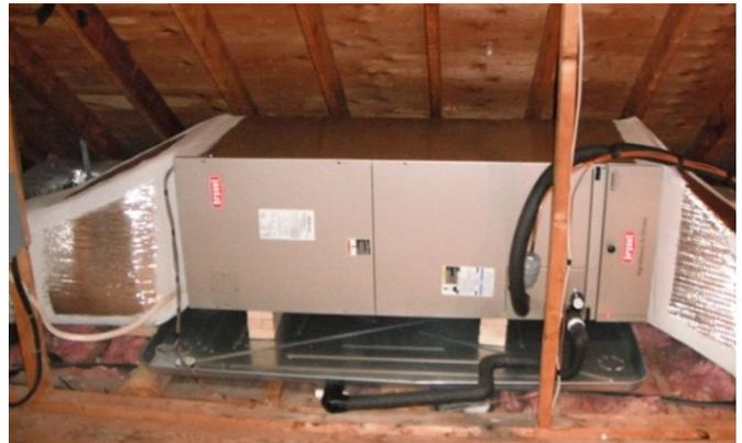
*Figure 4 - Ducted split system - indoor air handling unit.*
