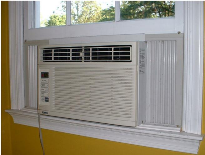
*Figure 2 - Packaged window air conditioning unit.*
