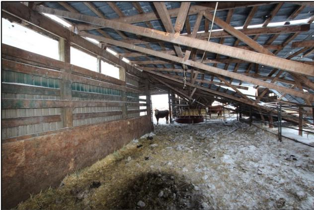
**Figure 10-** Example of roof collapse for a cattle barn contributed by corroded connector plates.
