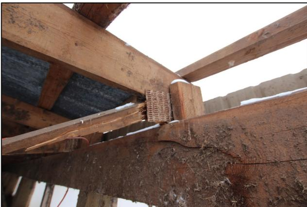
**Figure 11-** Example of a corroded connector plate in a collapsed roof.
