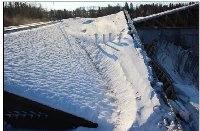
Figure 7- Example of snow accumulation in a roof valley.
