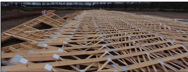
**Figure 1** - Roof collapse aftermath with neatly stacked trusses typically indicates inadequate or missing temporary roof/building bracing during erection.
