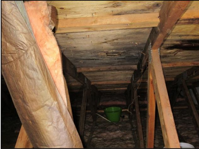
Figure 8- Decayed structural components in the attic due to poor roof waterproofing.
