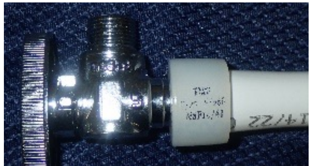
Barb not fully seated into tubing
