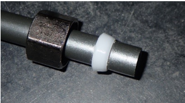
Insufficiently tightened fitting; ferrule loose, tubing will slip
