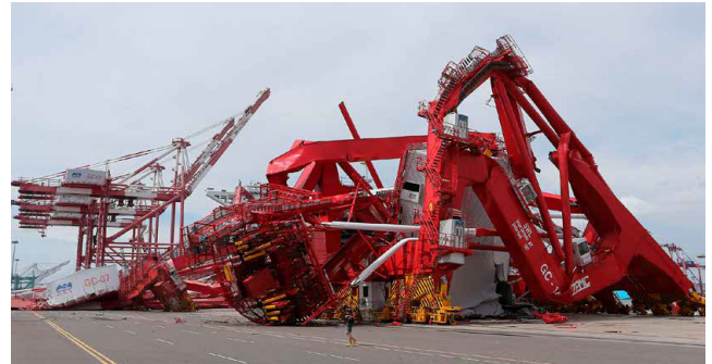
Figure 1A - Collapsed crane.
