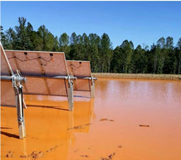
**Figure 3** - Flooding at a project site.
