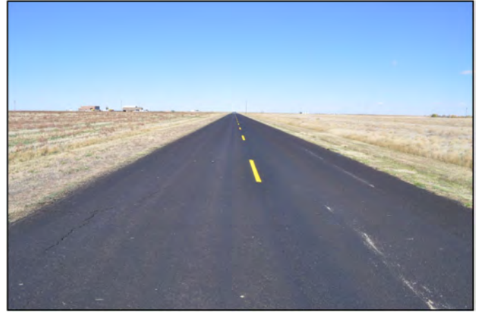
Figure 3. Test Site After Resurfacing
