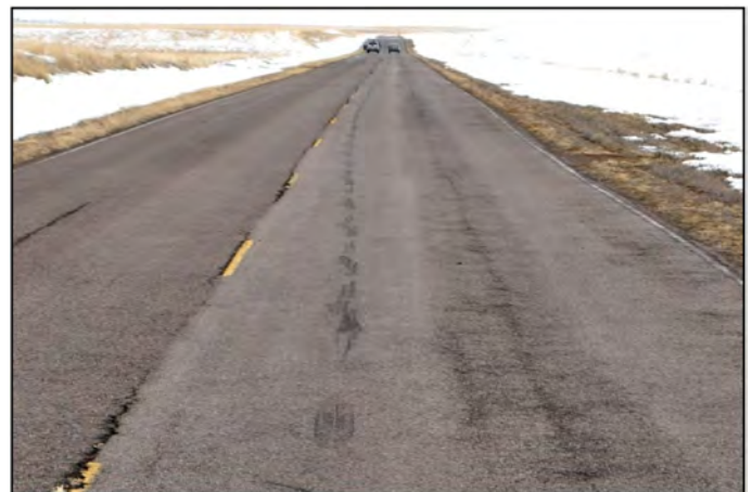
Figure 16. Tire mark from a partial tread separation
