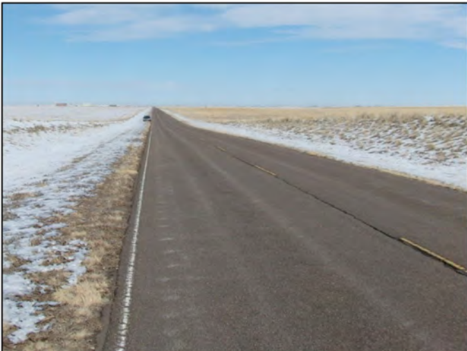
Figure 2. Test Site Prior to Resurfacing
